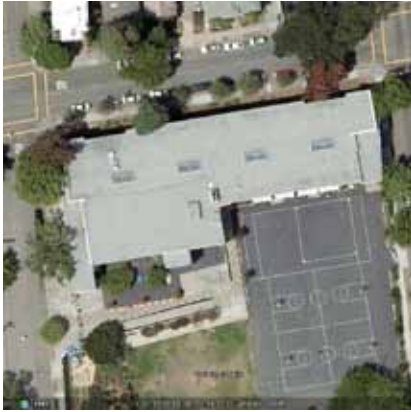
Washington Elementary in Berkeley, CA before solar installation.
